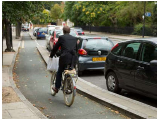
One-way cycle track with kerb segregation Source: TfL
