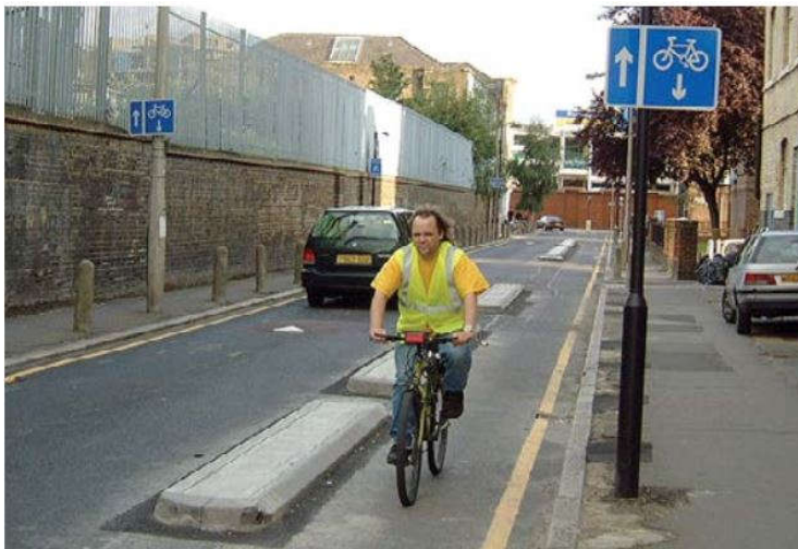
Contraflow with kerb island segregation
