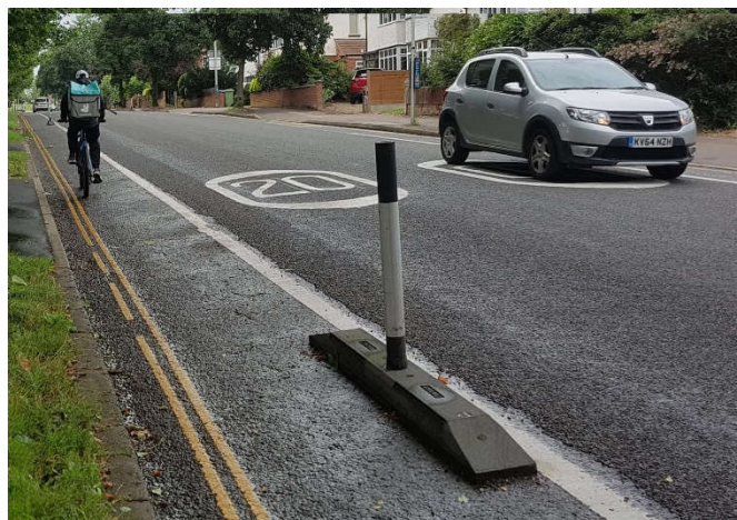
Mandatory cycle lane with light segregation Photo Credit: Derek, Norwich Cycling Campaign
