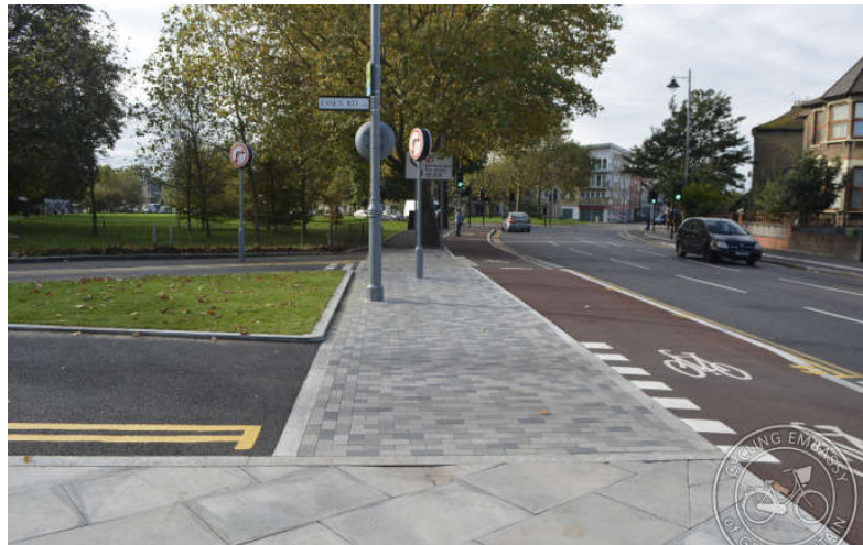
Continuous footway and stepped cycle track, Walthamstow
