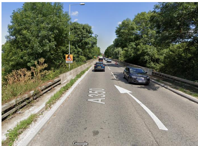
G) River Avon overbridge south of Farmers Roundabout (north)
