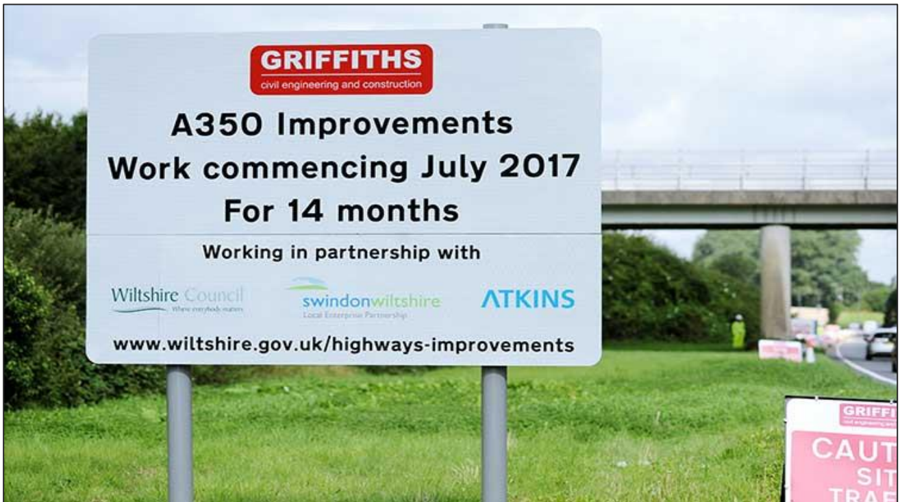
Figure 6-3 – A350 Badger Brook and Chequers Improvements, collaborative delivery
