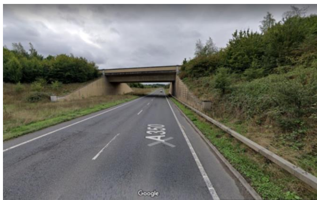
J) Kennet and Avon Canal Aqueduct (south)
