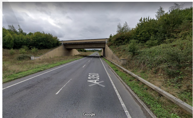
J) Kennet and Avon Canal Aqueduct (south)
