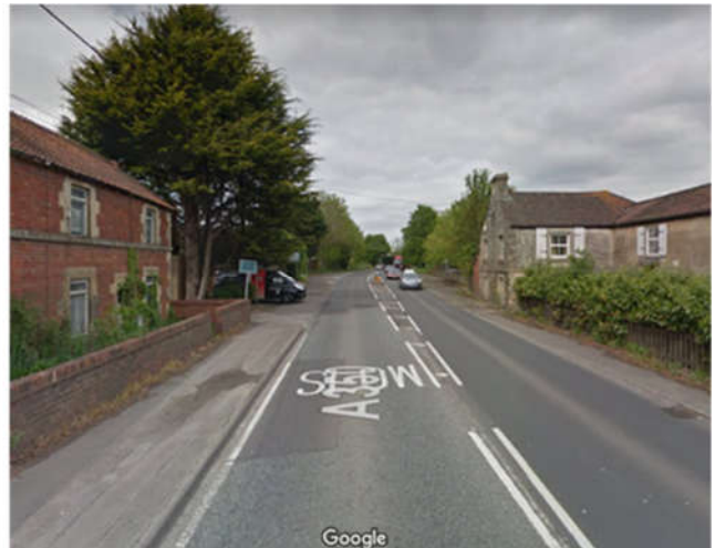
B) South of Westlands Lane Junction
