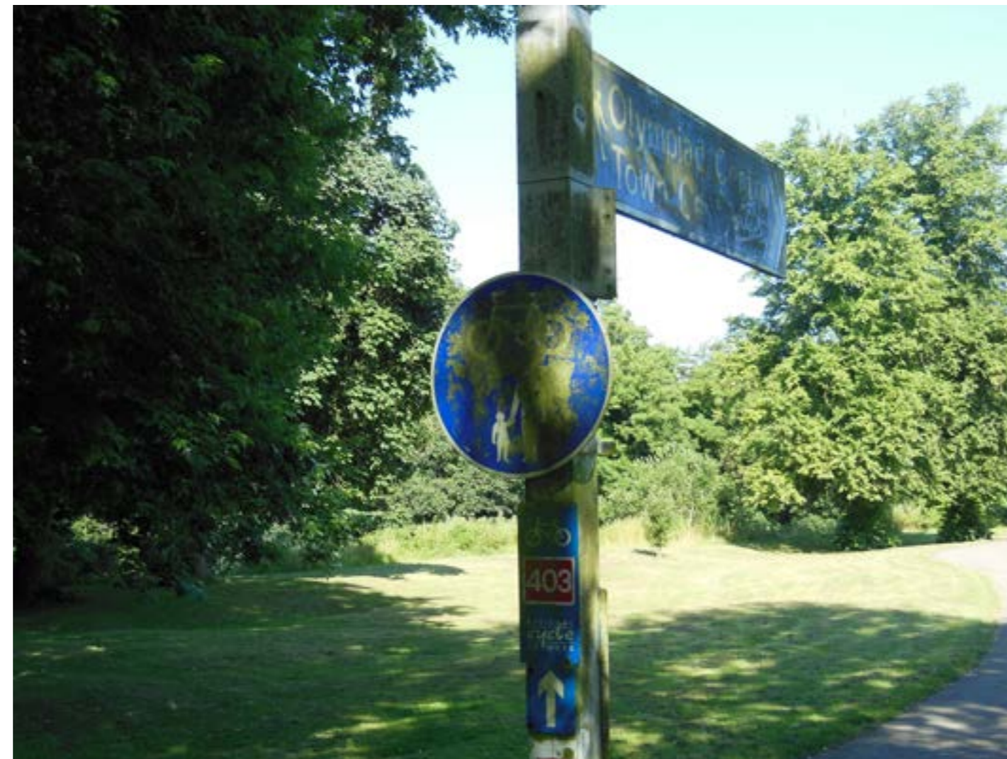
In damp, wind-beaten settings, materials are more prone to weathering and regular maintenance is essential, especially for DfT signage.
