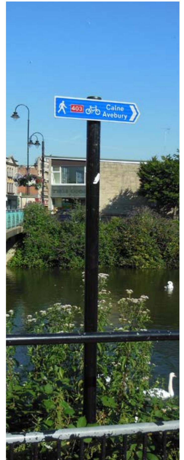
Context sensitive design is important; this sign could have been mounted on the railing to reduce clutter.
