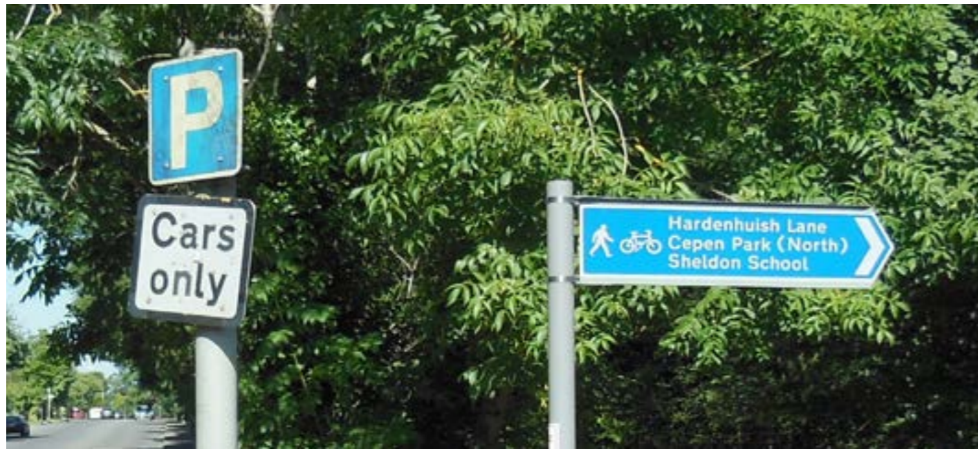
Signage positioned in close proximity could be rationalised onto a single pole to reduce clutter and maintenance costs going forward.
