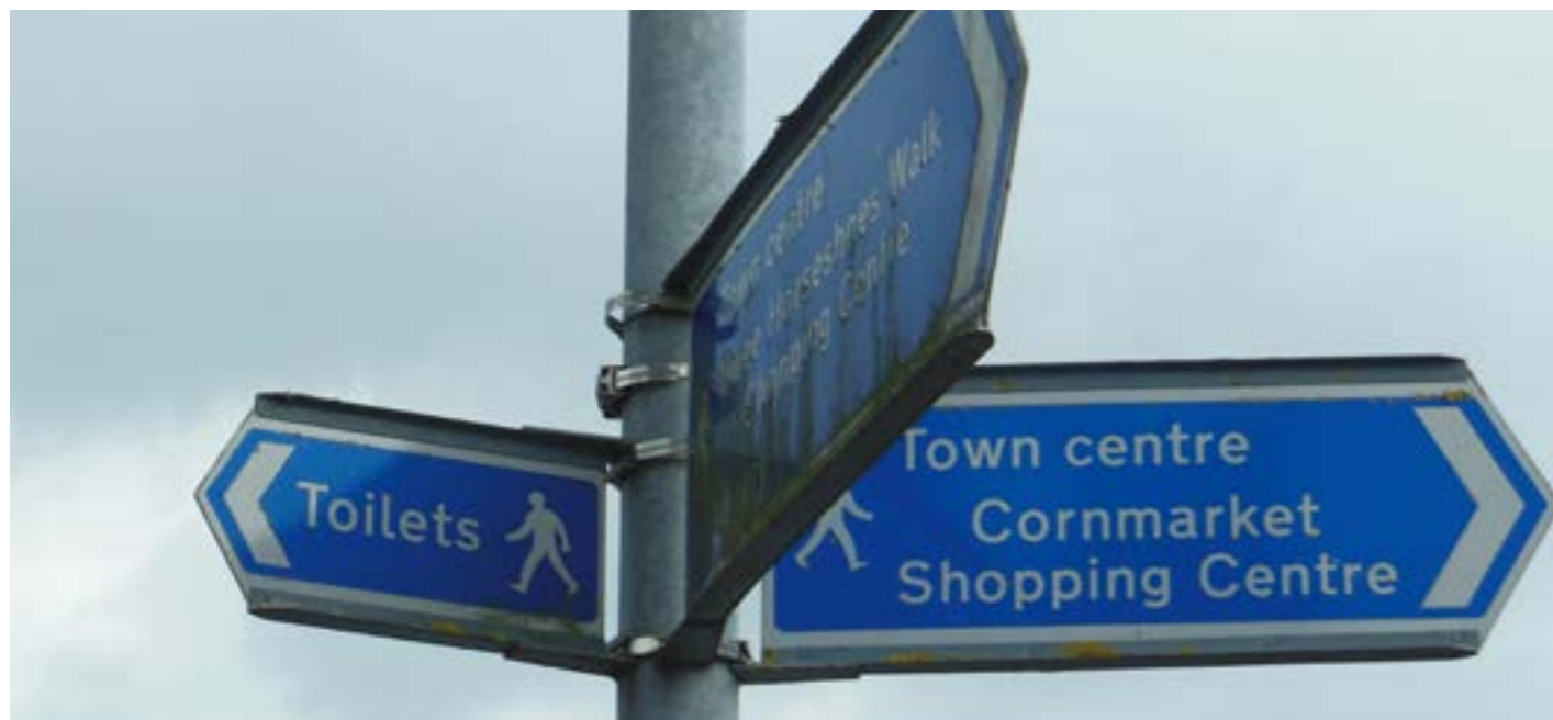
TSRGD direction signs for pedestrians are generally clear and concise, but in need of maintenance.
