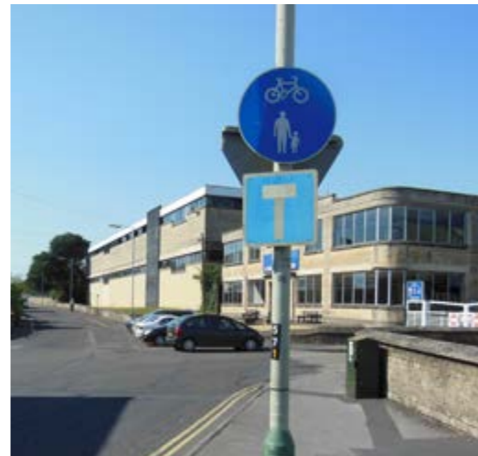
Using existing posts and lamp columns is an effective way of putting up new signage if needed.
