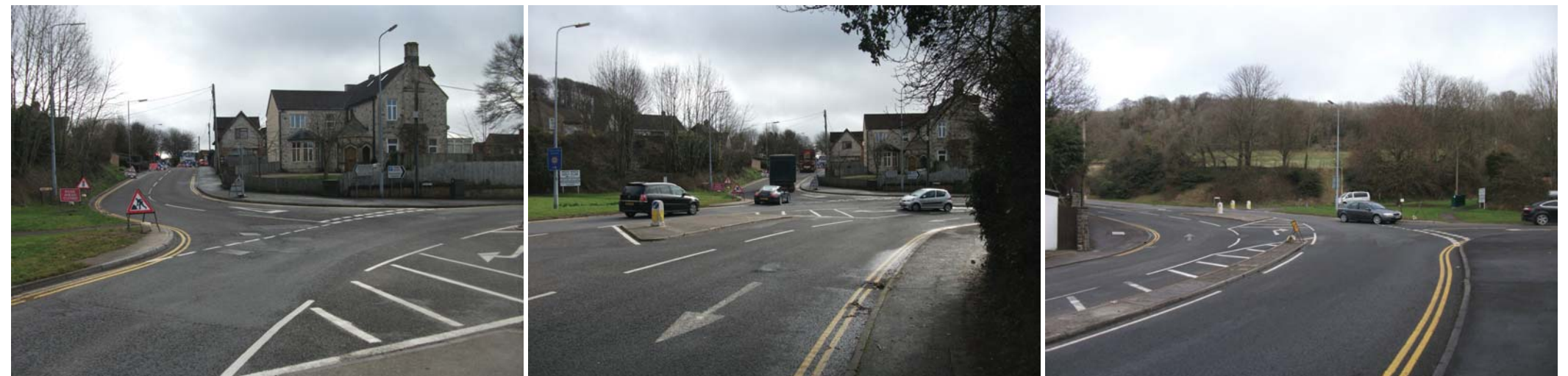
Proposed sign location - existing conditions
