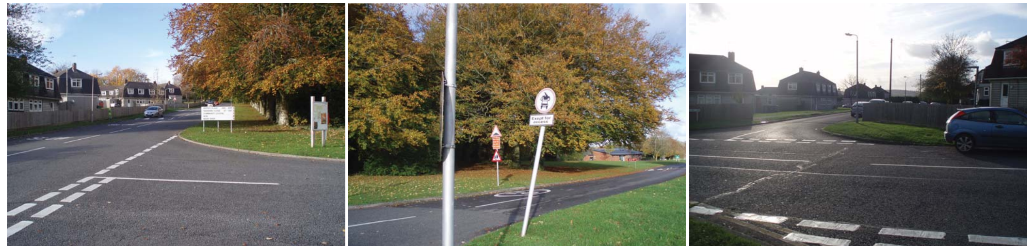
Proposed sign location - existing conditions
