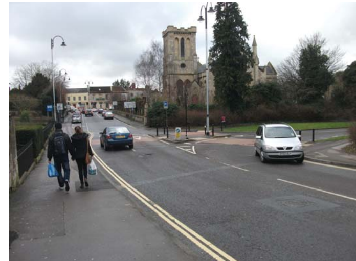
Proposed sign location - existing conditions
