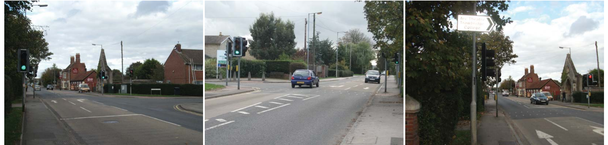
Proposed sign location - existing conditions
