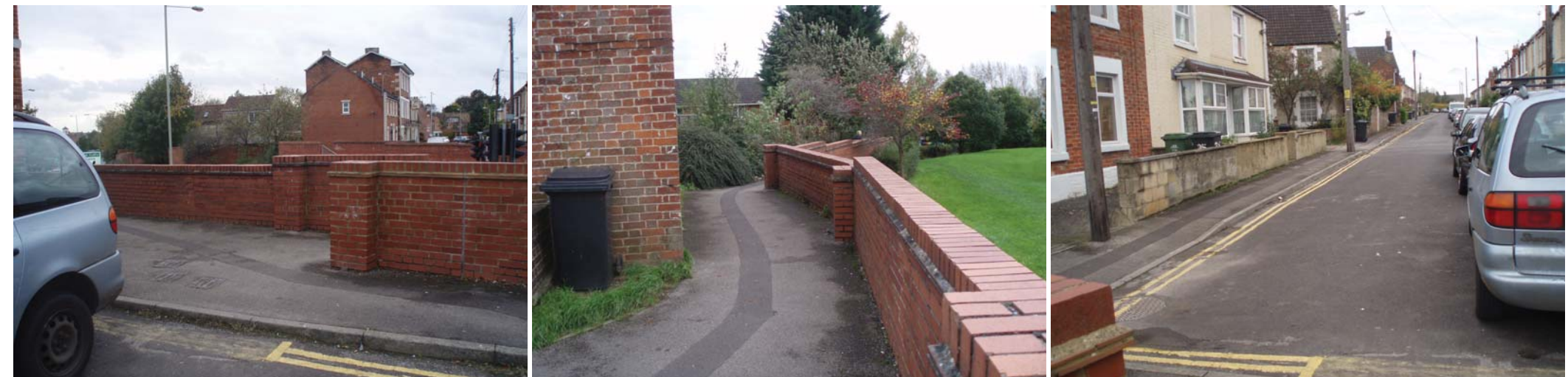
Proposed sign location - existing conditions
