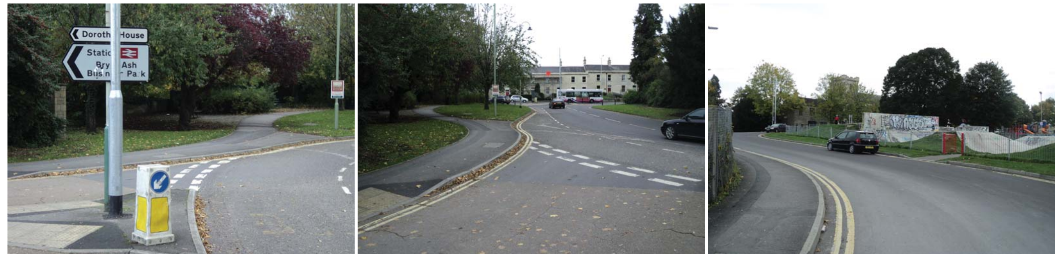
Proposed sign location - existing conditions
