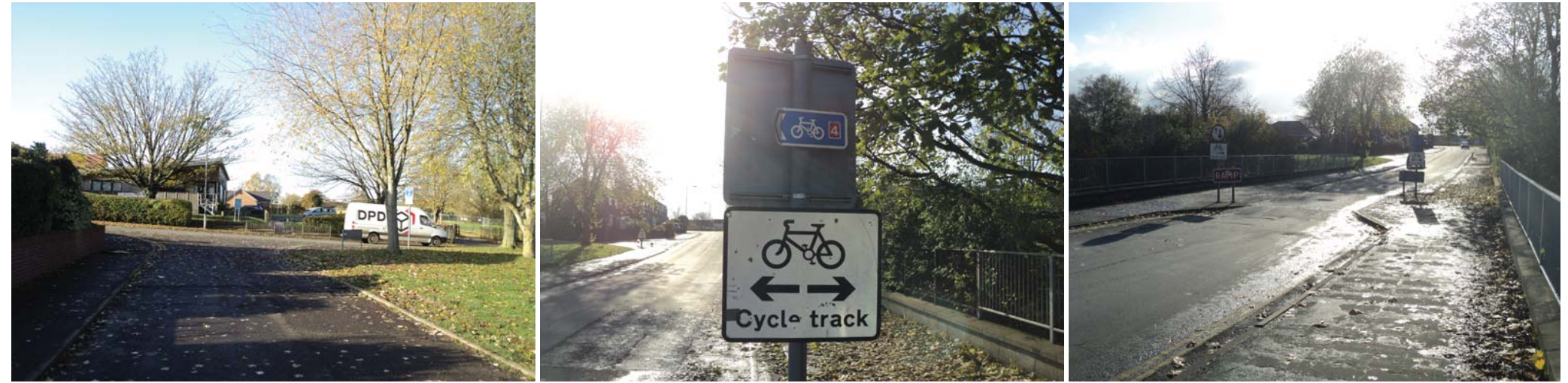
Proposed sign location - existing conditions
