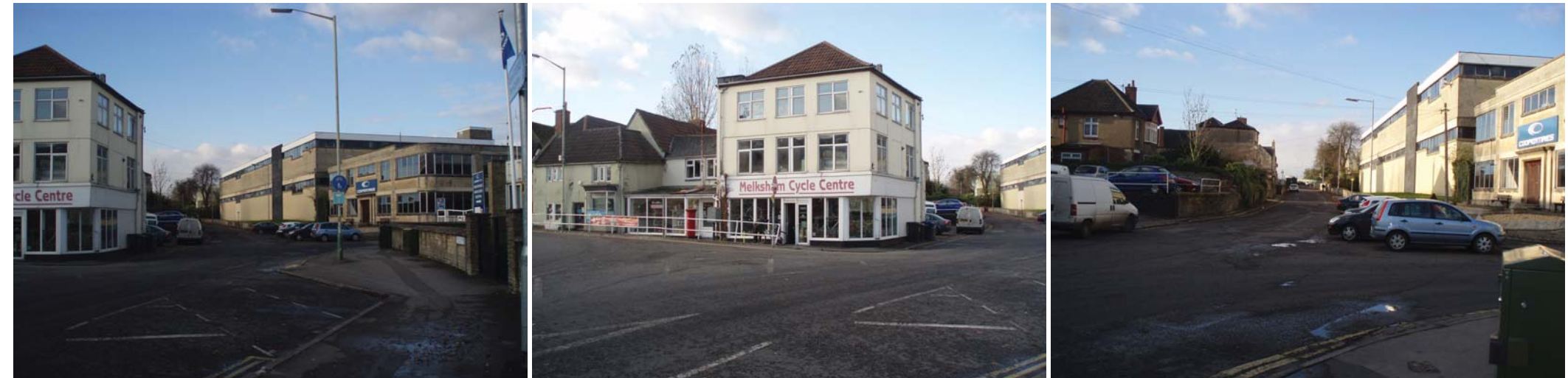
Proposed sign location - existing conditions
