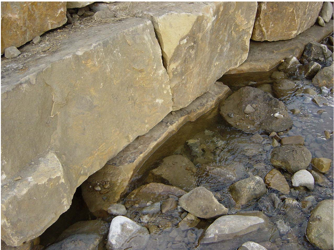
Detail of reinforced bank showing new submerged crevices and reinstated channel
