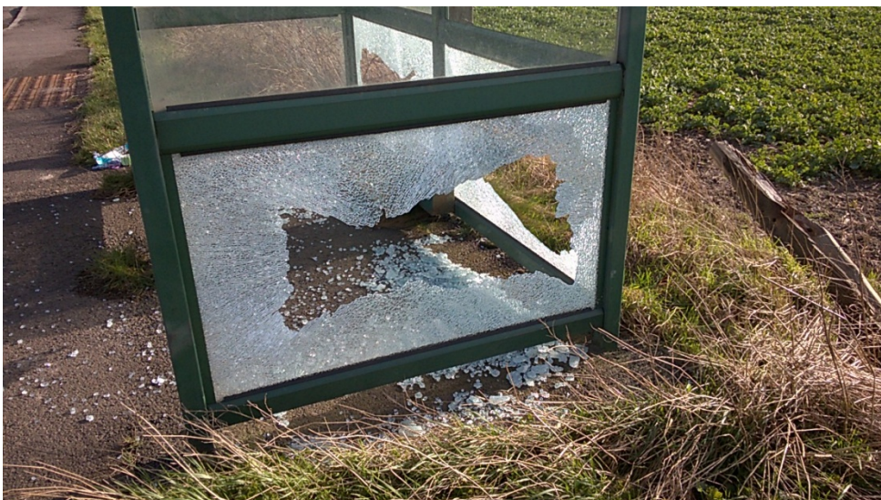
Damaged with Broken Glass or Sharp Edges (BRGL)
