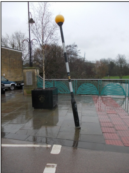
Damaged electrical installations and equipment (LIGH)
