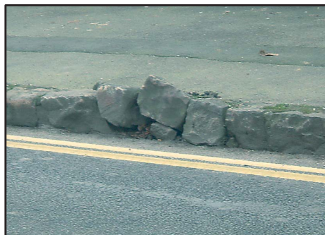
Kerb vertical projection, damaged or missing (EVPJ, DAMG, MISS)
