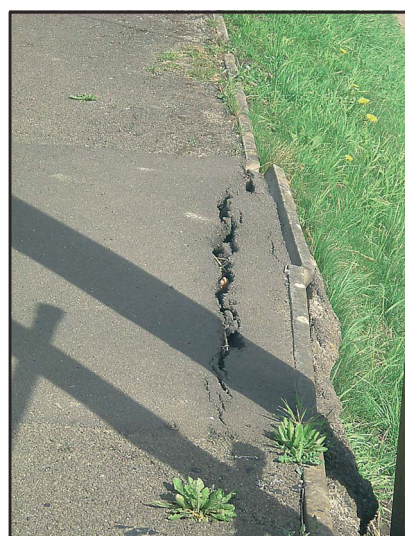
Footway cracks and gaps (MACK)
