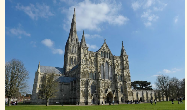
Salisbury Cathedral and City, 1 of 3 'Principal Settlements'
