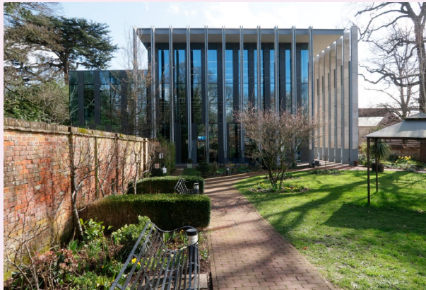
Bourne Hill Council Offices, Salisbury
