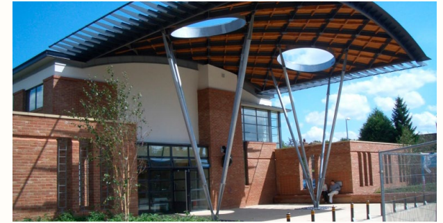
Wiltshire Police Station, Trowbridge
