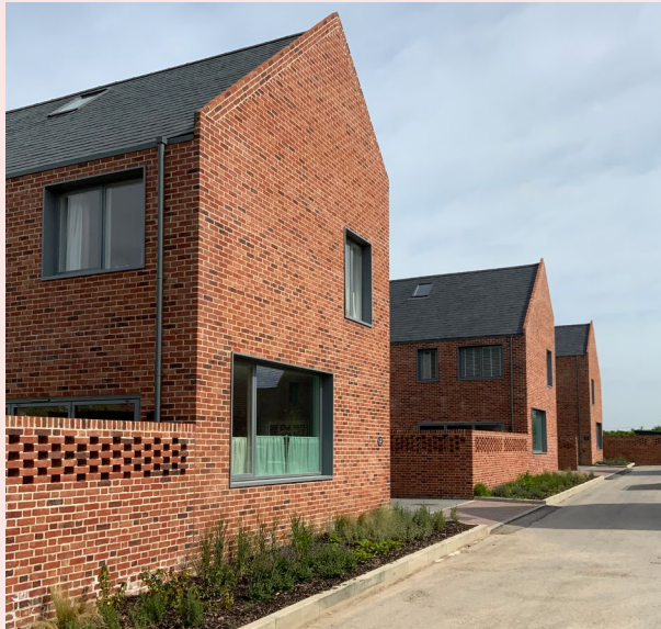
Side gables include large windows to habitable rooms. Boundary walls include perforated brickwork. The Tannery, Holt.
