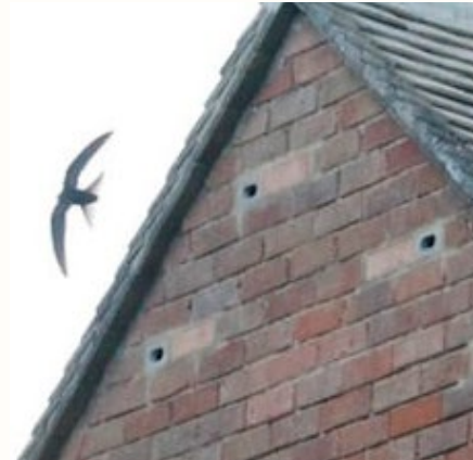
'Universal bricks' integrated within the building's fabric.
