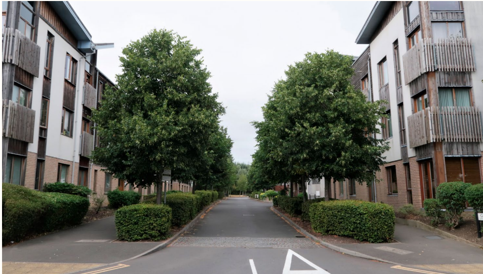
Distinctive boulevard enclosed with 3 storey housing, Great Mead, Chippenham
