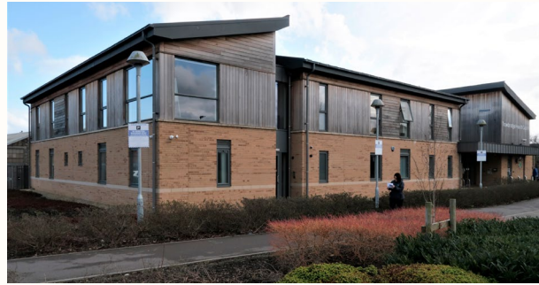
Trowbridge Health Centre
