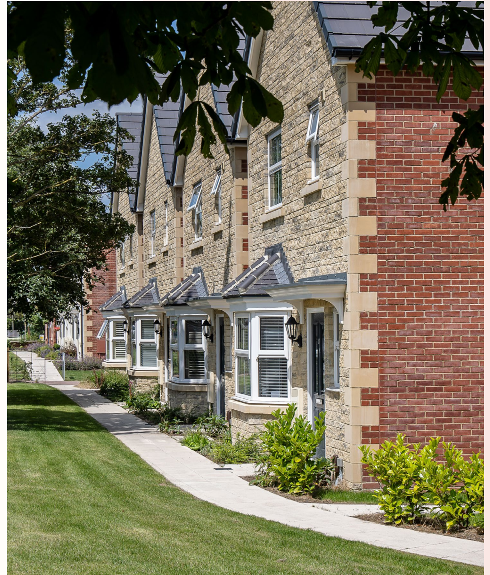
Newland Place, Trowbridge
