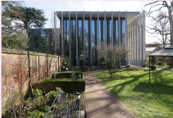
Bourne Hill Council Offices, Salisbury
