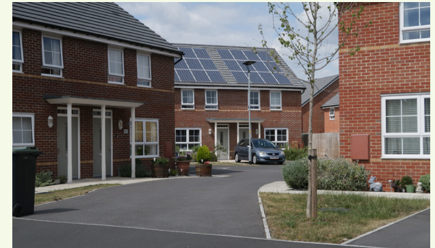
Owner-installed solar panels on south facing roof of new housing, Sandridge Place, Melksham
