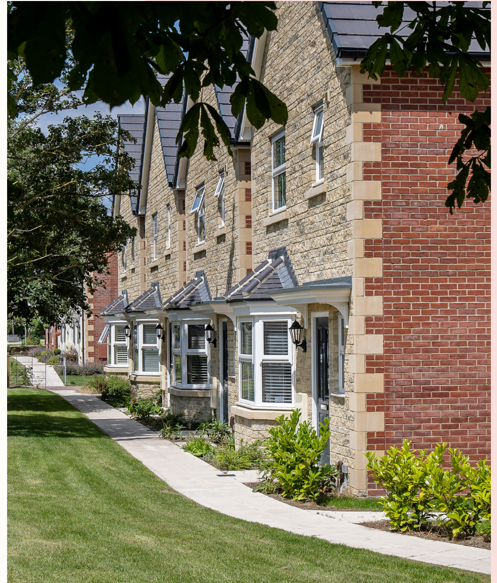
Newland Place, Trowbridge
