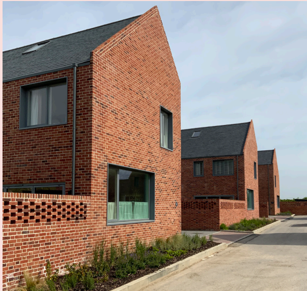
Side gables include large windows to habitable rooms. Boundary walls include perforated brickwork. The Tannery, Holt.
