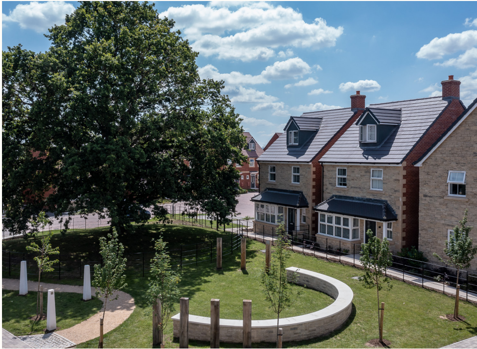
Newland Place, Trowbridge
