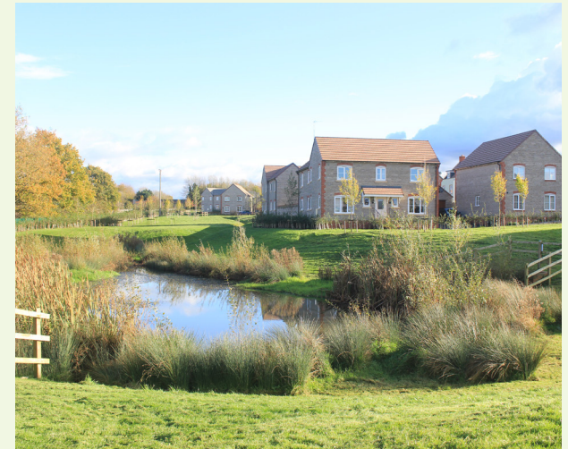
SuDS designed as a natural pond with accessible, split level banks, Ridgeway Farm, Purton Parish, Wiltshire
