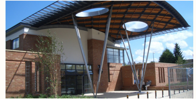
Wiltshire Police Station, Trowbridge
