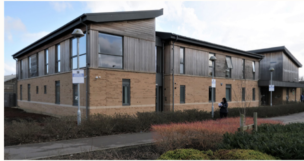
Trowbridge Health Centre
