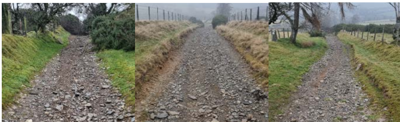
Photo: The condition of the road along sections that have not been purposefully damaged to prevent motorised access. It is quite clear decades of motorised use since any maintenance work has taken place, has not caused any of the alleged 'destruction'.
