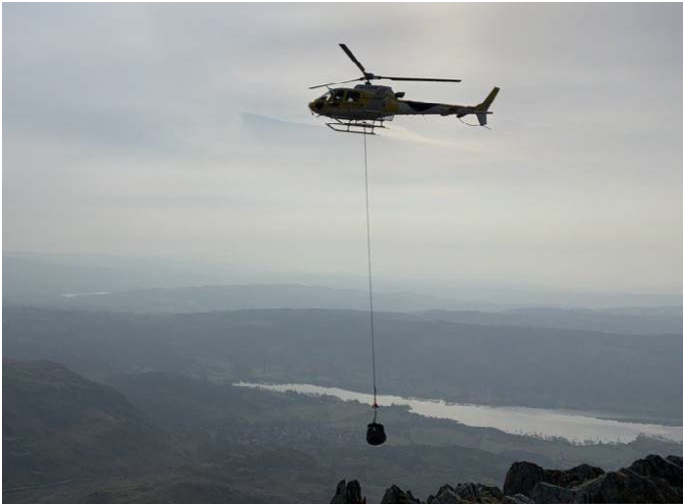
Photo: A helicopter used to transport stones to a path on Coniston Old man (Pic: Fix the Fells)
