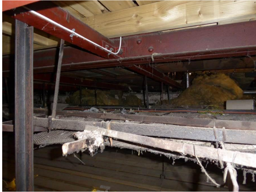
Photo 21 – Historic ceiling substructure.
