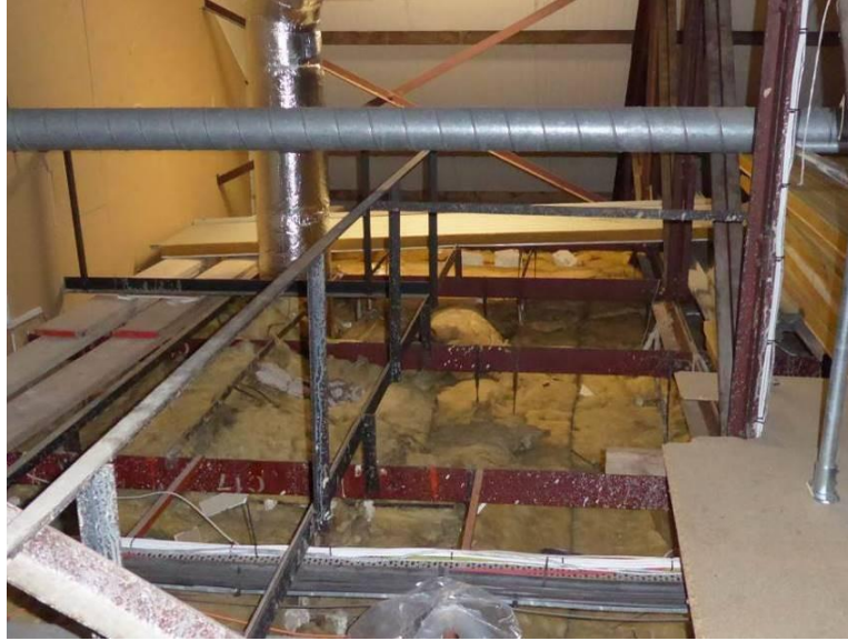
Photo 29 – Ceiling above Alamein Room.
