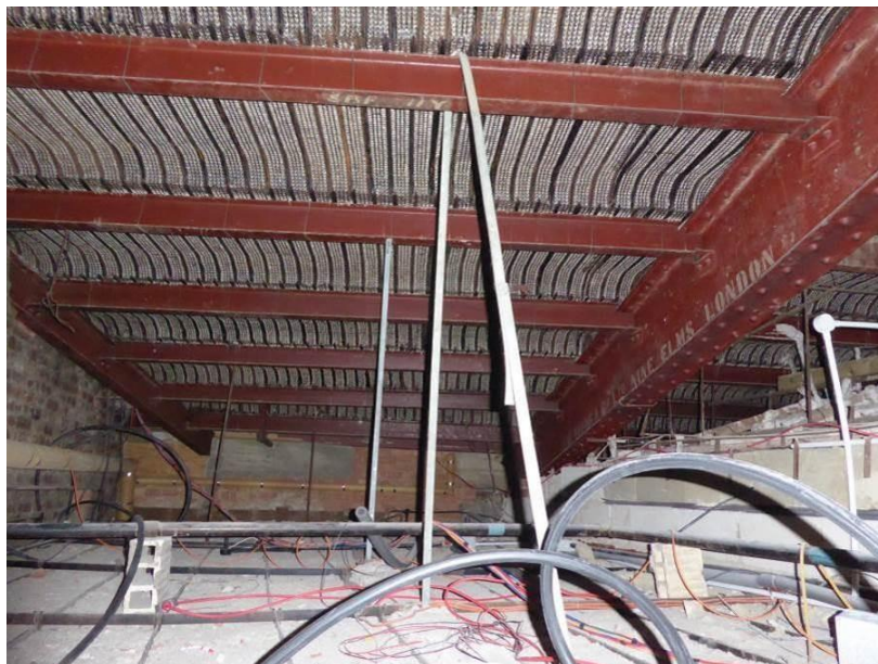
Photo 8 – ceiling void above Kitchen / Servery.
