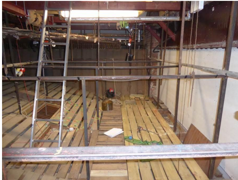
Photograph A1.17 – Lighting platform over Auditorium, next to stage.
