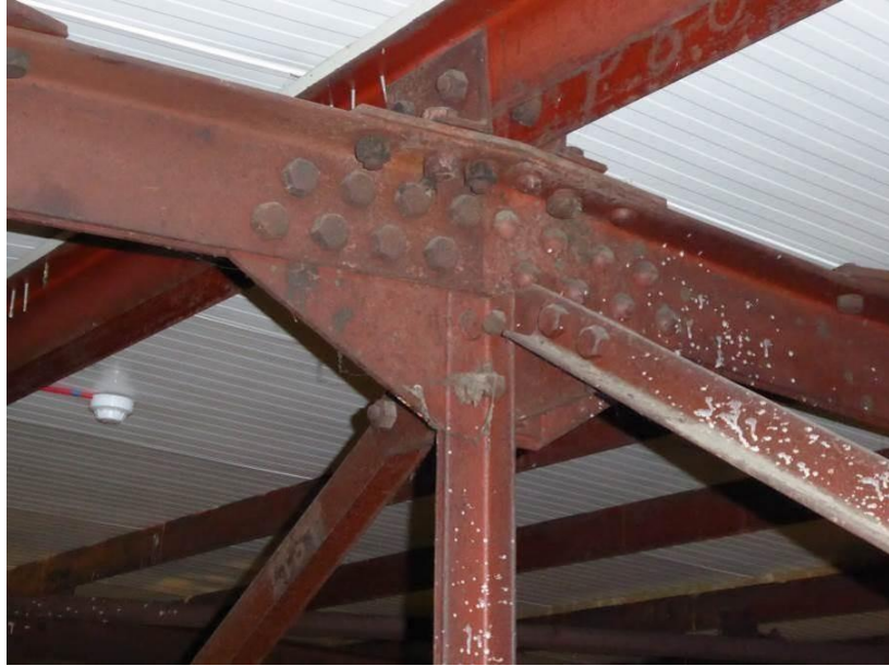
Photo 13 – Truss connection.
