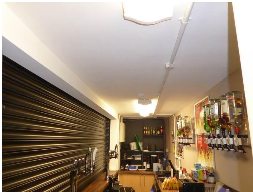
Photos 8 and 9 – Ceilings over the Servery and the Kitchen.
