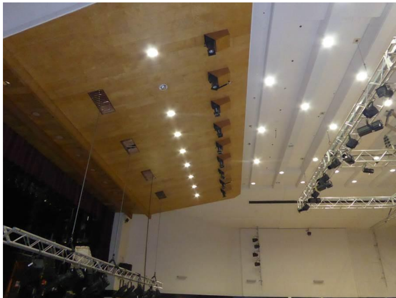
Photo 22 – Lighting platform, underside view.
