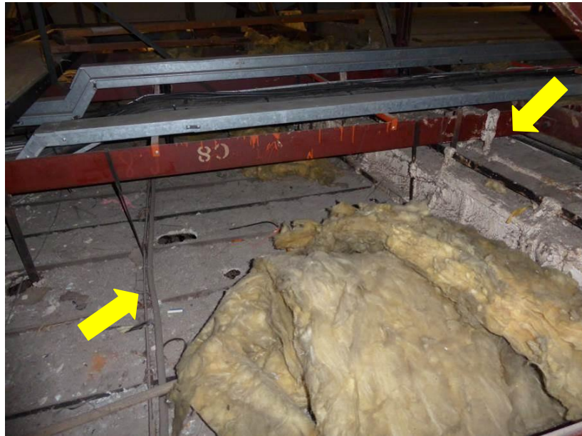
Photo 19 – Suspended ceiling, visible junction with high level ceiling.
