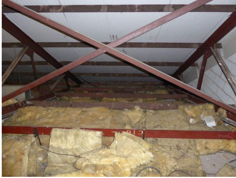
Photo 18 – Void over vaulted ceiling.
