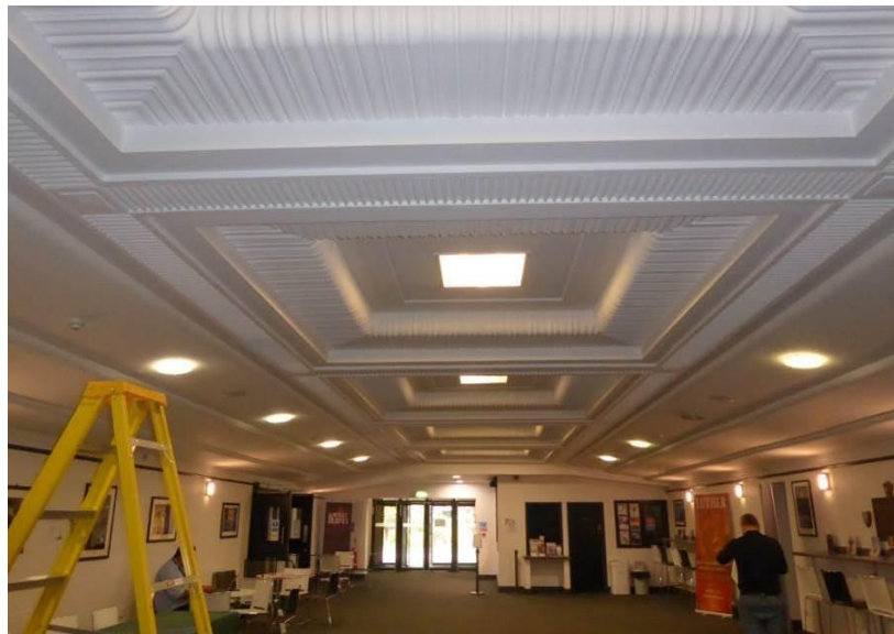
Photo 4 – The suspended ceiling over Foyer.
