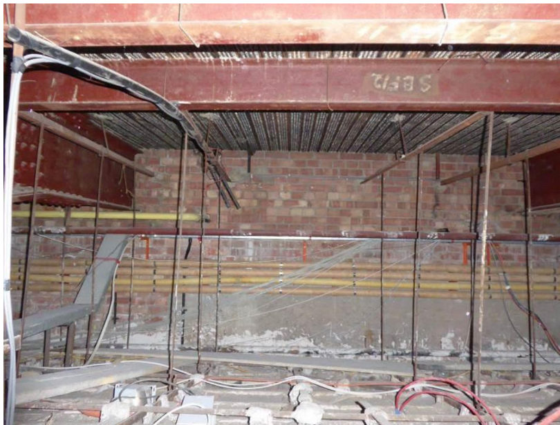
Photograph A1.14 – Ceiling void over Foyer.
