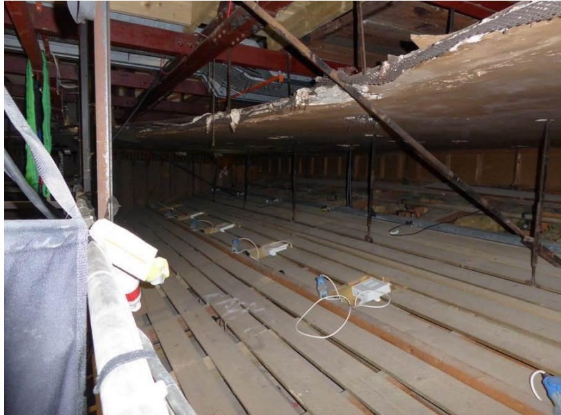
Photo 21 – Suspension of the lighting platform.
