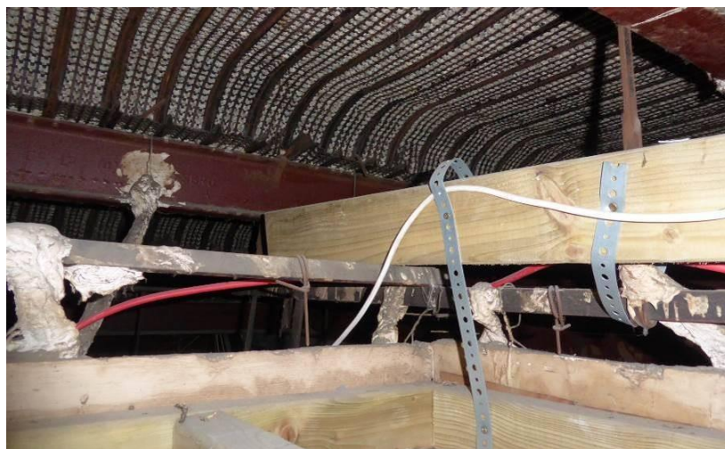
Photo 5 – Timber frame around light fitting, over the coffer.
