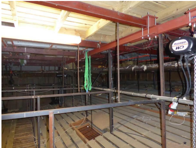
Photo 20 – Steel subframe supporting lighting platform.
