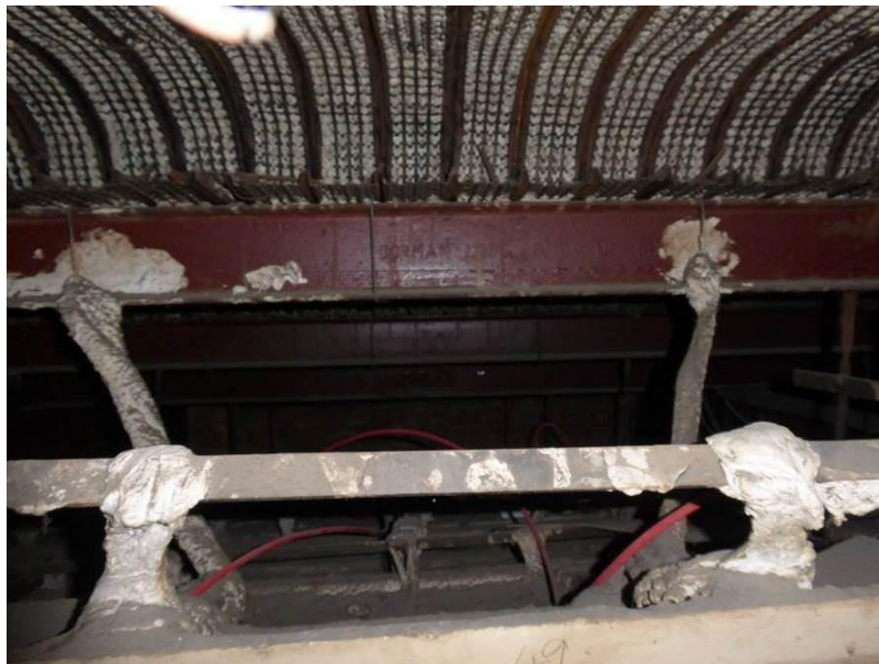
Photo 3 – Hessian wadding ties supporting the suspended ceiling.
