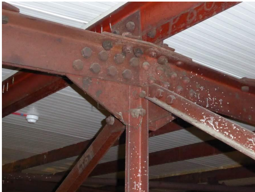
Photo 12 – Truss connection.
