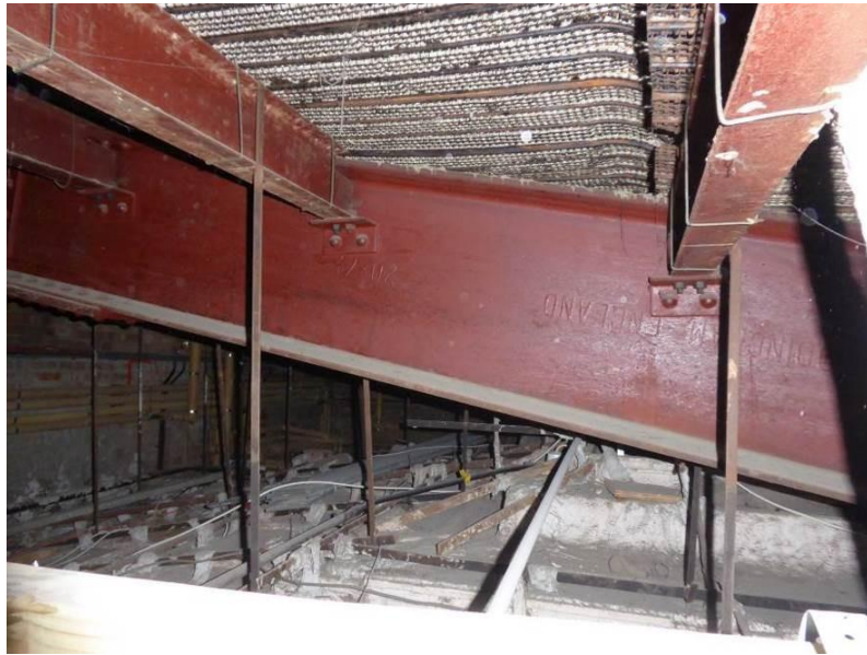
Photo 1 – Ceiling void above Foyer.
