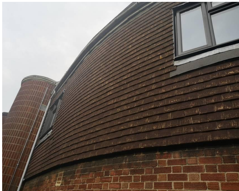
Photograph A2.14 – Part tile hun east elevation. Note tiles and some of the brickwork have been painted with a non-breathable coating.
