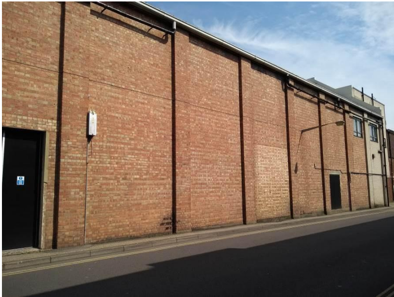
Photograph A1.6 – West elevation, central part to side of auditorium.
