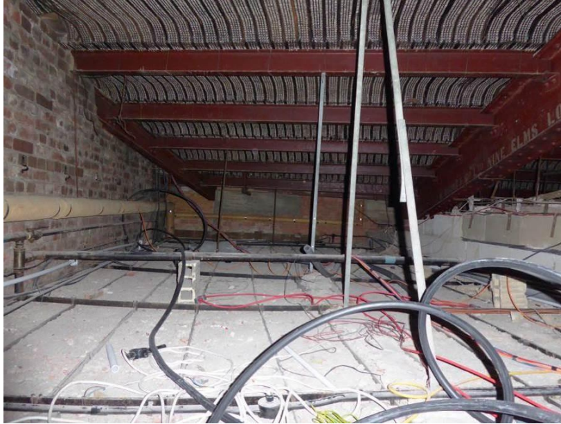
Photograph A1.13 – Ceiling void over Kitchen / Servery.
