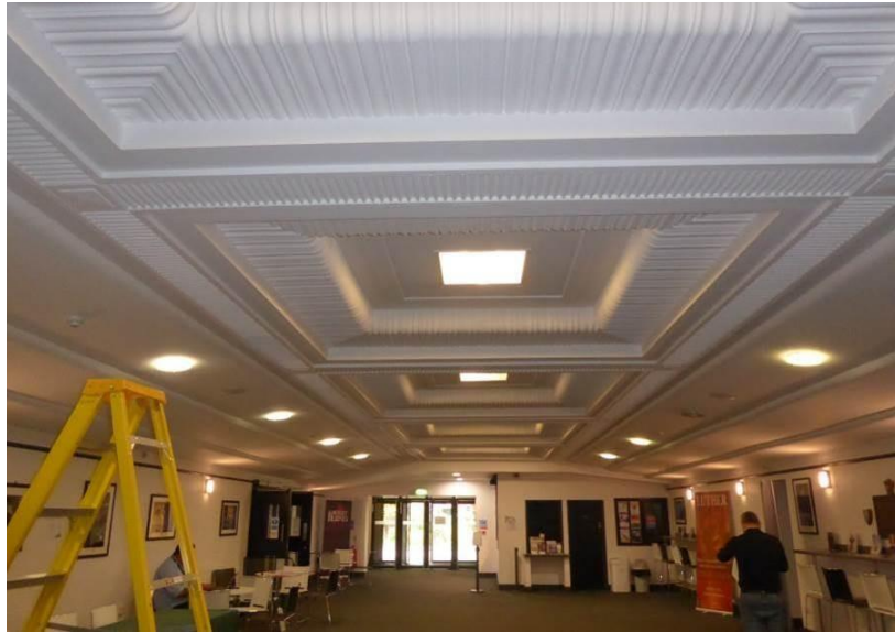
Photo 4 – The suspended ceiling over Foyer.
