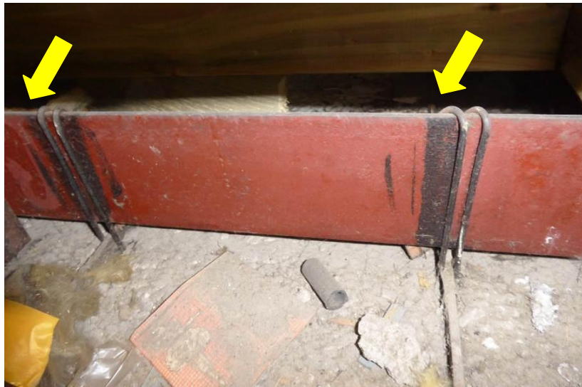
Photo 16 – Metal wire ties fixing flat bars to the angle.
