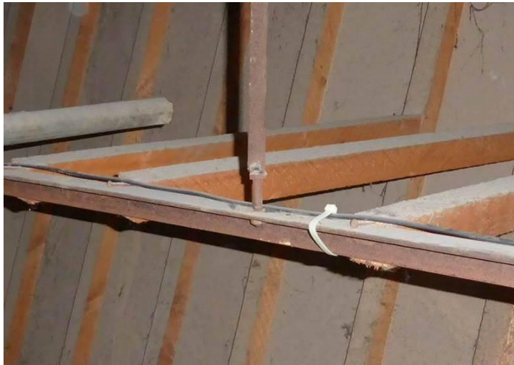
Photo 34 – Tie connection in the lighting platform's suspension system.
