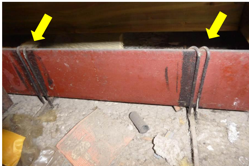
Photo 18 – Metal wire ties fixing flat bars to the angle.
