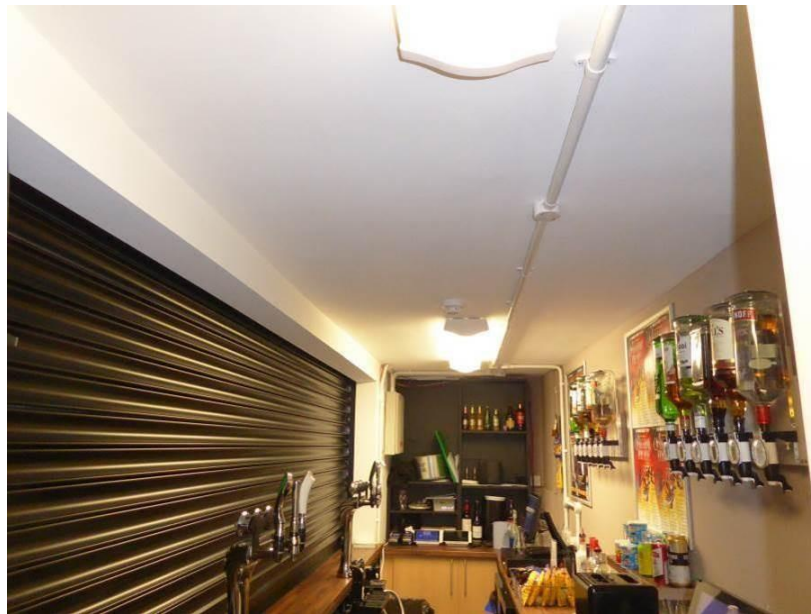
Photograph A1.10 – Kitchen servery ceiling.
