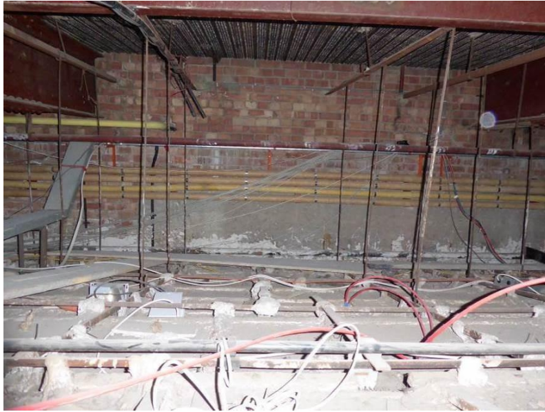
Photo 2 – Ceiling void above Foyer.
