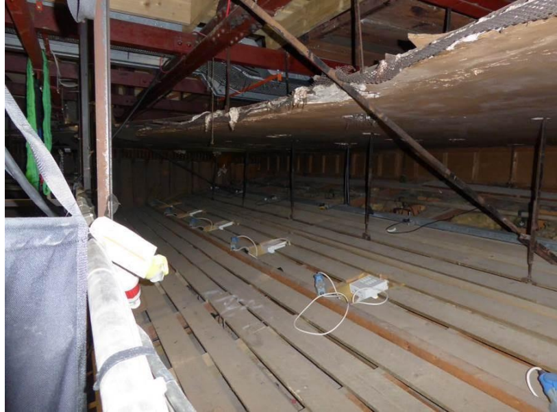
Photo 23 – Suspension of the lighting rig.
