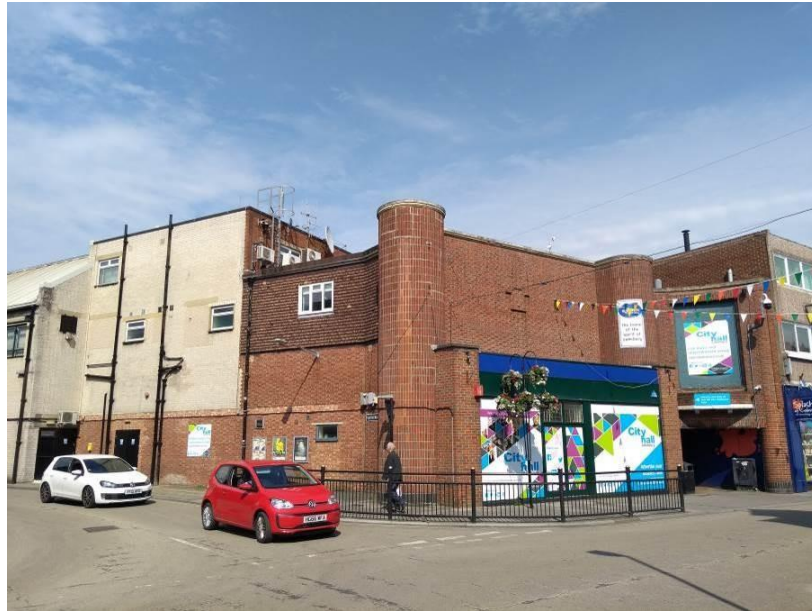
Photograph A1.7 – Front / South elevation.
