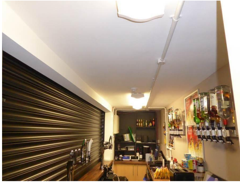
Photo 10 – Ceiling over the Servery.
