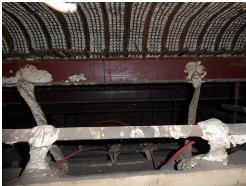
Photo 3 – Hessian wadding ties supporting the suspended ceiling.
