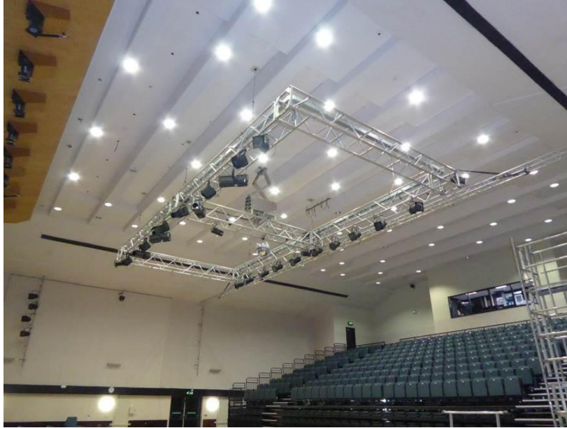
Photo 23 – Ceiling over the Auditorium.
