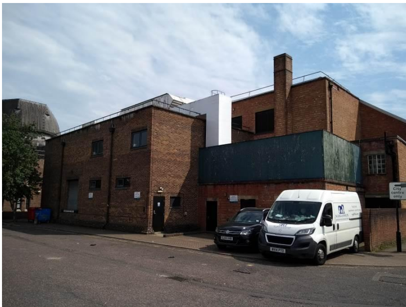
Photograph A1.4 – North elevation.
