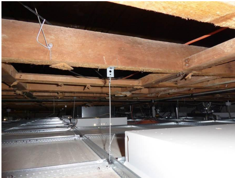
Photo 31 – Tiled suspended ceiling and timber frame over Alamein Room.
