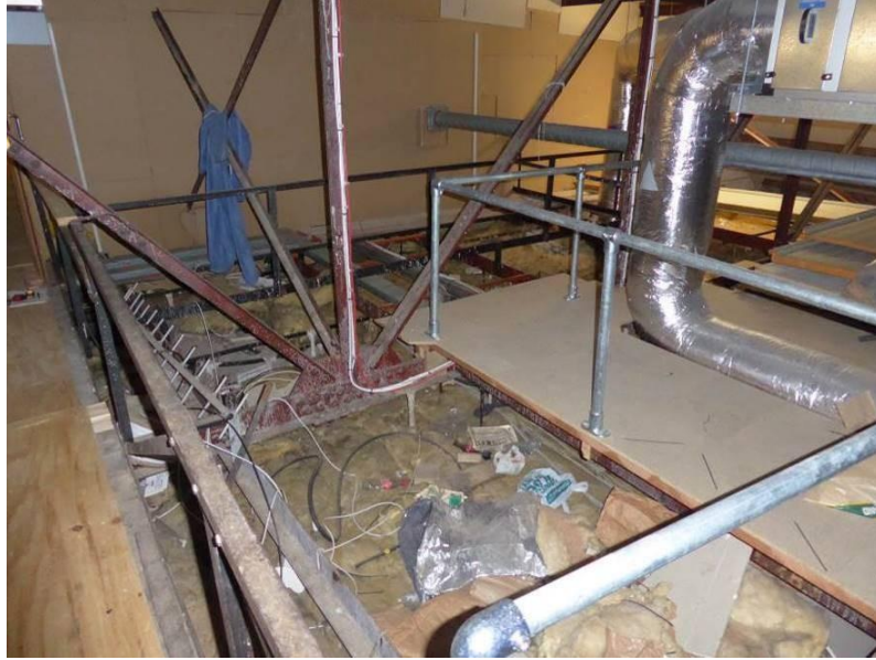
Photo 28 – Loft above Alamein Room.
