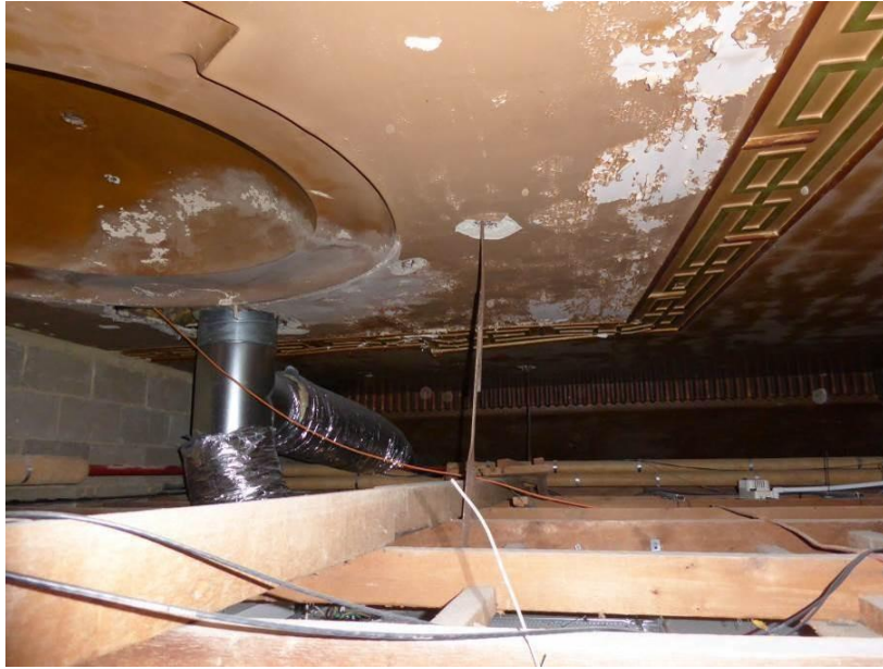
Photo 30 – The underside of suspended ceiling over Alamein Room.
