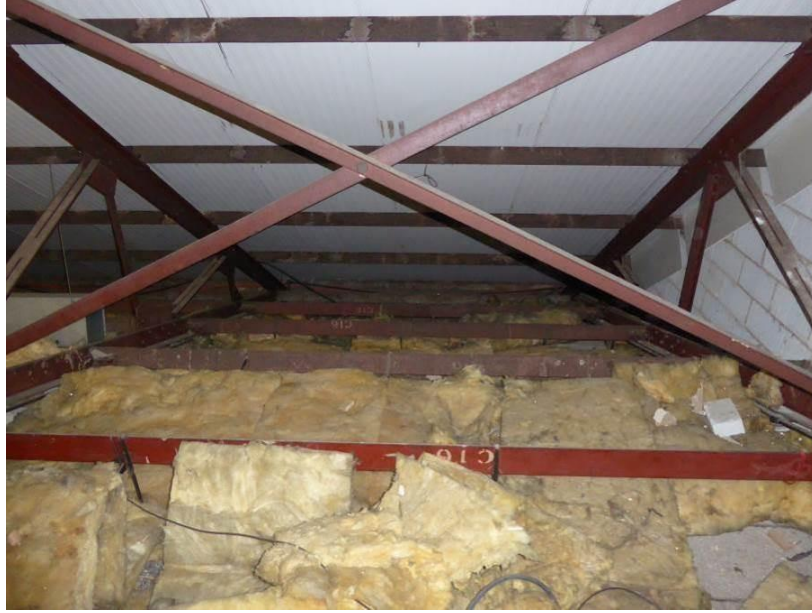
Photo 20 – Void over vaulted ceiling.
