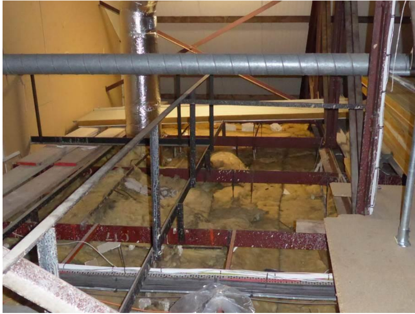
Photo 27 – Ceiling above Alamein Room.
