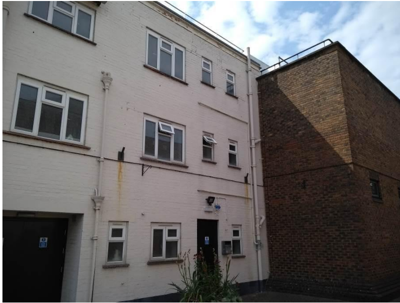
Photograph A1.3 – East elevation (North end).
