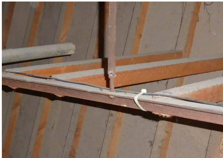
Photo 31 – Tie connection in the lighting platform's suspension system.
