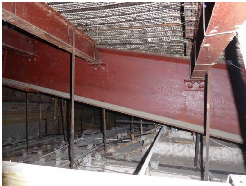
Photo 1 – Ceiling void above Foyer.
