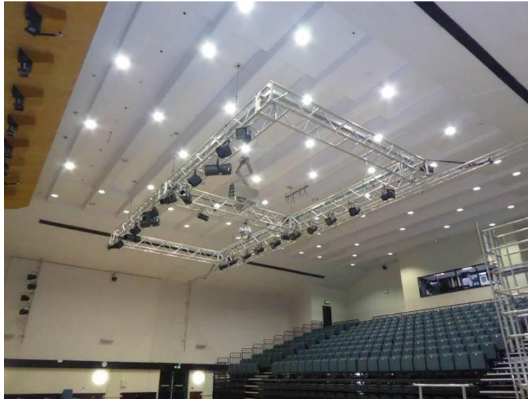
Photo 25 – Ceiling over the Auditorium.
