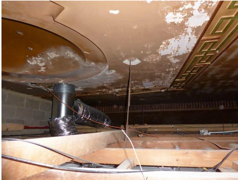
Photograph A1.19 – Original ceiling above in the Alamein Room.
