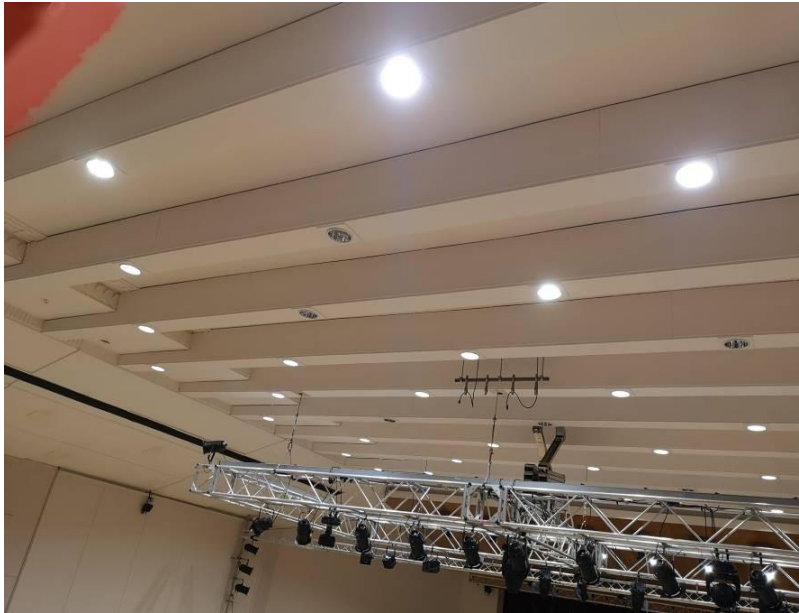
Photograph A3.1 – Main auditorium ceiling on third visit.
