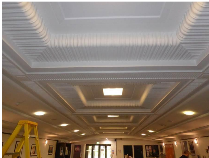
Photograph A1.8 – Foyer ceiling general view.
