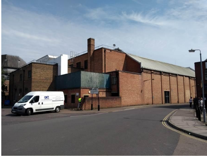
Photograph A1.5 – West elevation, North end.
