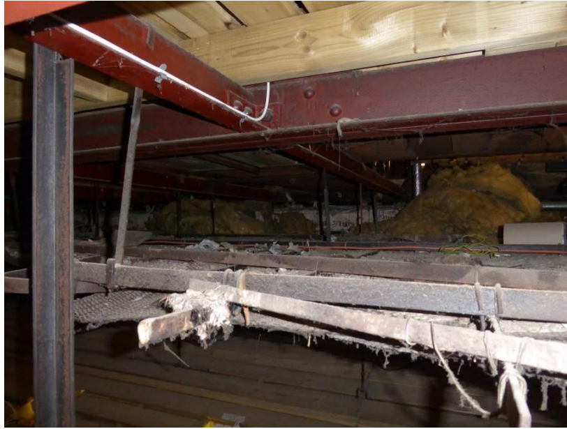
Photo 19 – Historic ceiling substructure.
