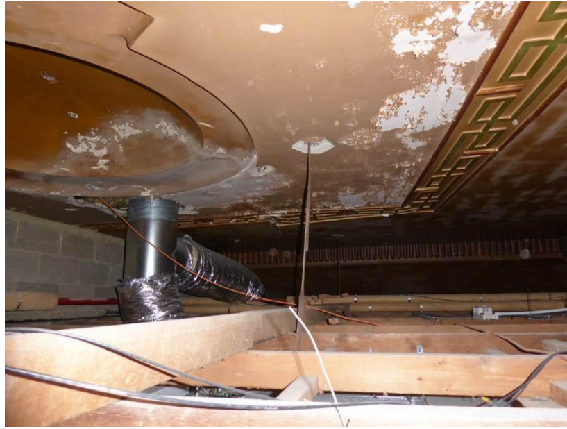
Photo 32 – The underside of suspended ceiling over Alamein Room.
