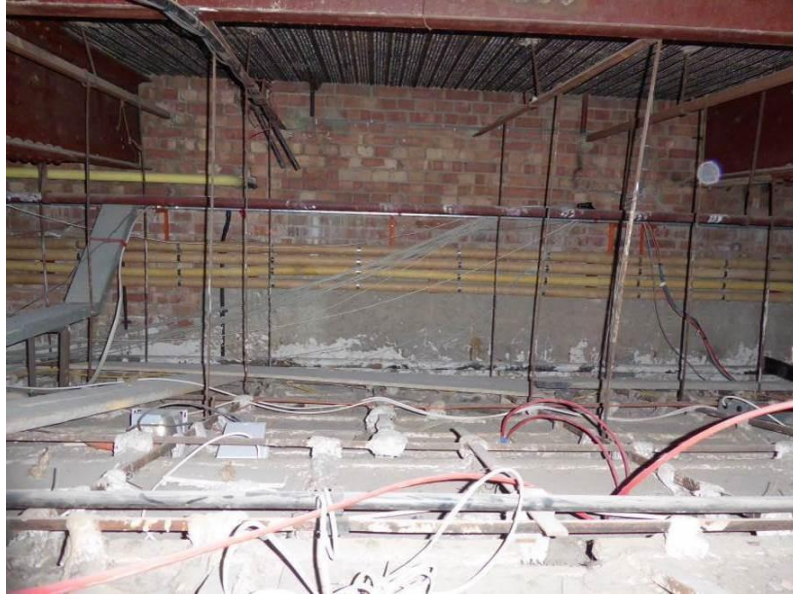
Photo 2 – Ceiling void above Foyer.
