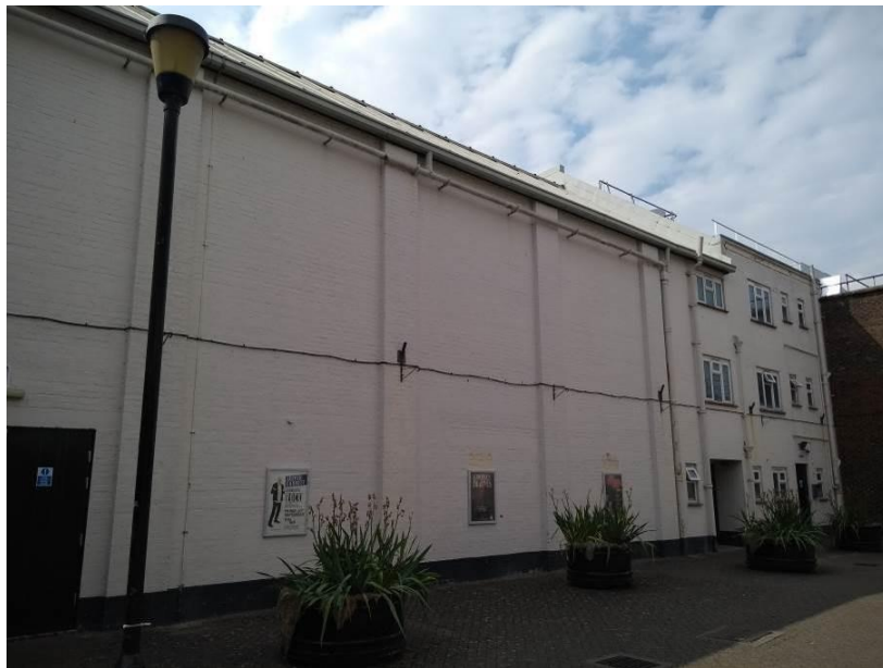
Photograph A1.2– East / side elevation, auditorium external wall.
