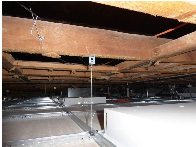
Photo 33 – Tiled suspended ceiling and timber frame over Alamein Room.
