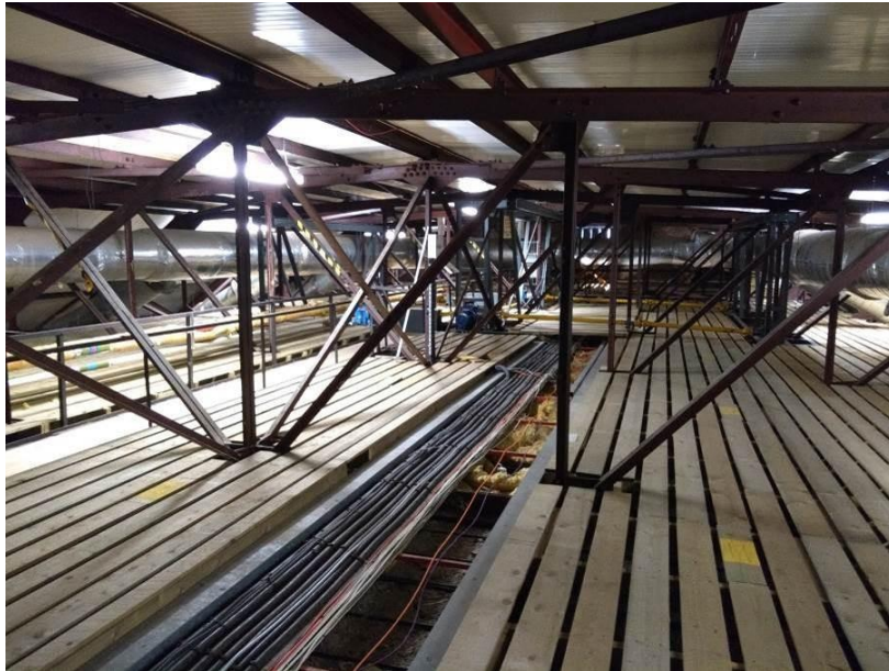
Photograph A1.15 – Loft over auditorium, general view.
