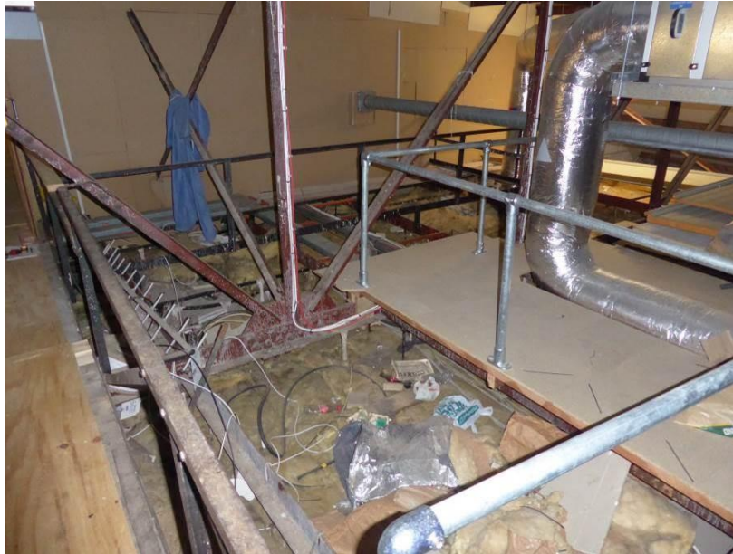
Photo 26 – Loft above Alamein Room.
