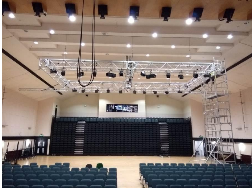
Photo 11 – Auditorium, retractable seating and lighting rig.
