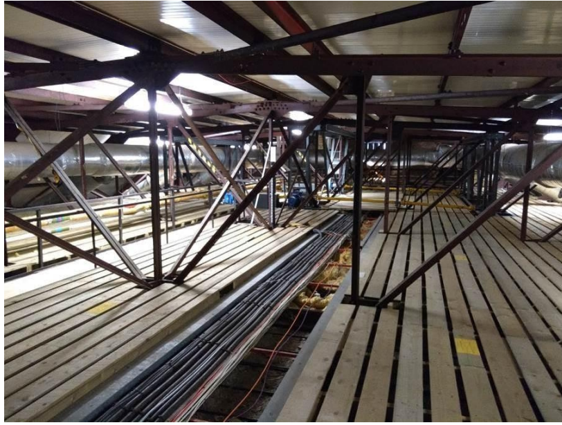
Photo 11 – Loft above Auditorium.
