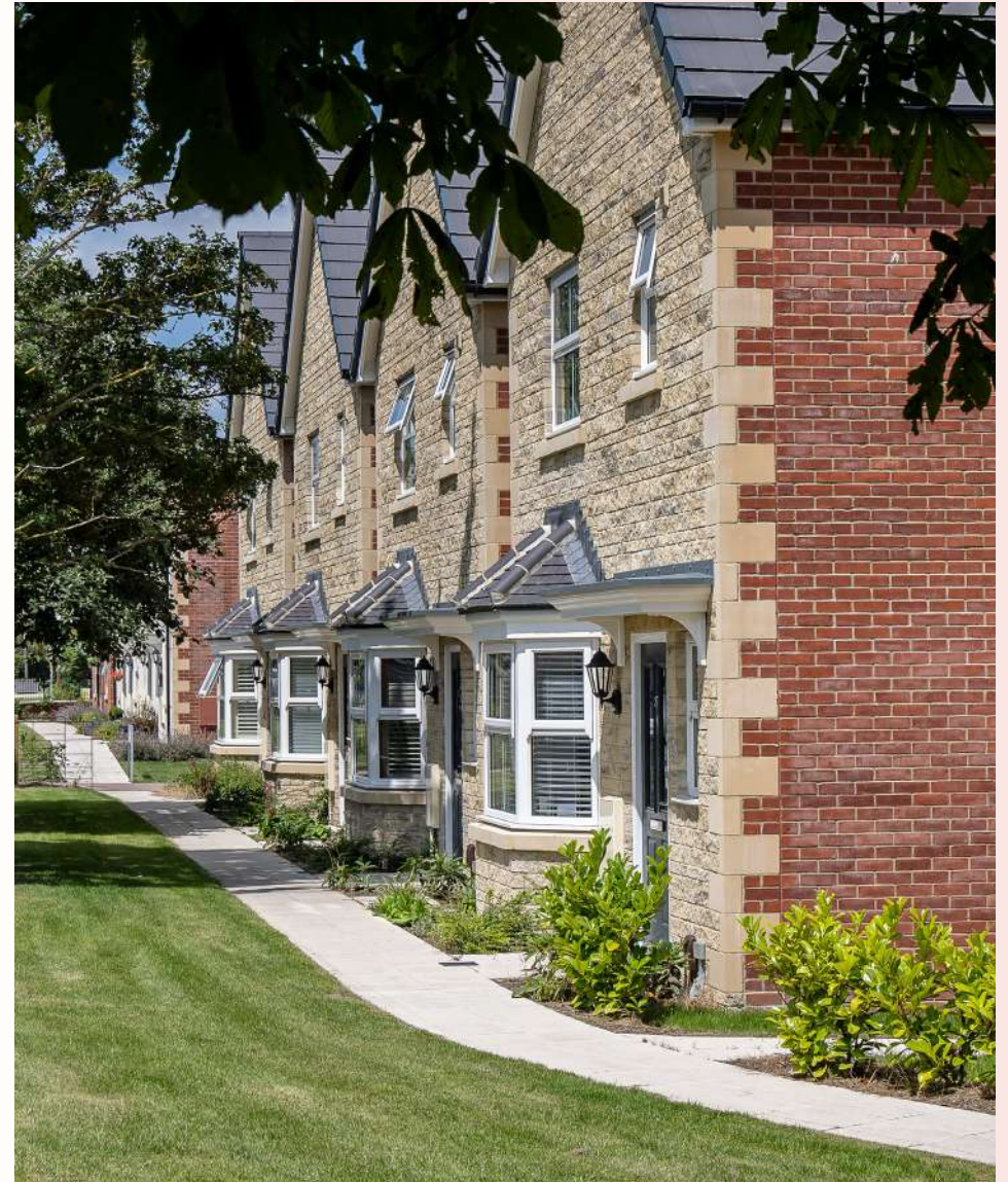
Newland Place, Trowbridge
