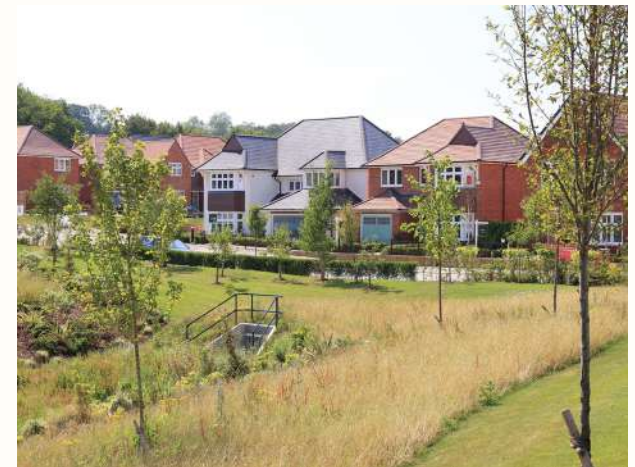
Generously planted Sustainable Drainage Systems within Marleberg Grange, Marlborough
