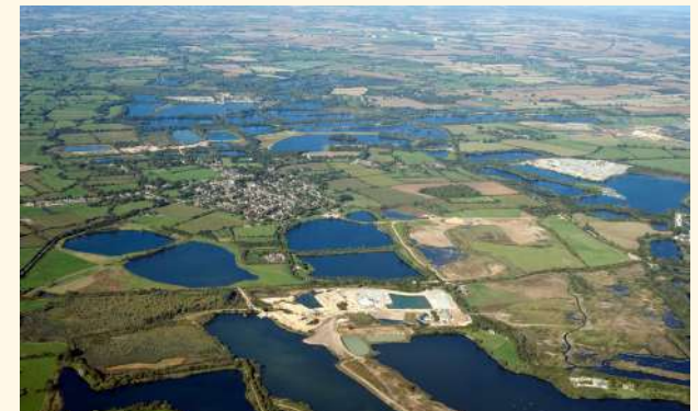
The Cotswold Water Park. A distinctive landscape of over 140 manmade lakes created from decades of mining. It continues to be a changing landscape with expanding recreational resource for the county and its visitors. Photo by Robert Bewley (copyright).
