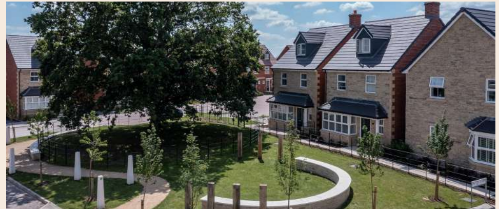
Newland Place, Trowbridge
