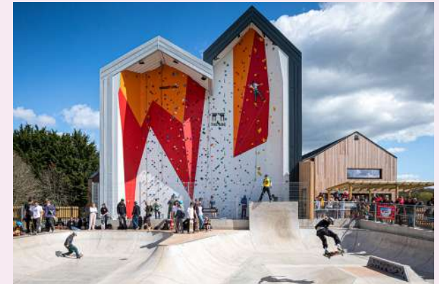
The Arc Climbing Academy, Chippenham, Photo by Paul Twomey (copyright).
