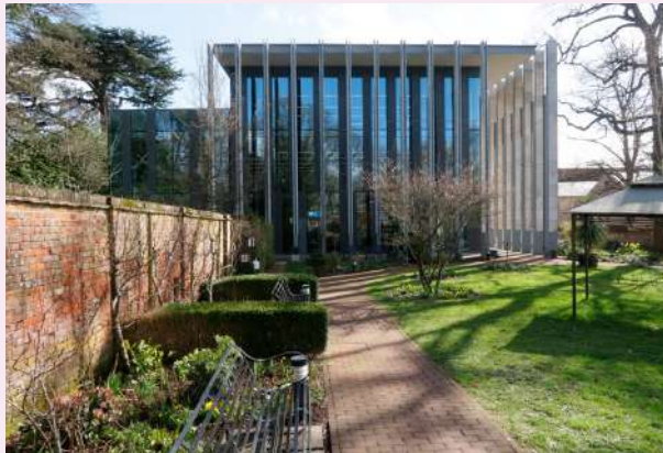
Bourne Hill Council Offices, Salisbury
