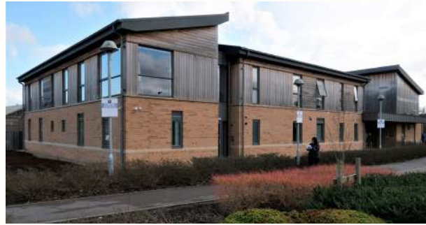
Trowbridge Health Centre
