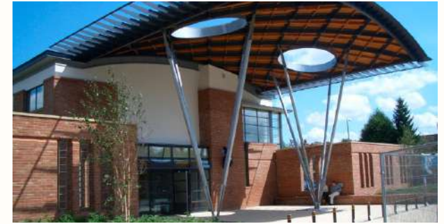
Wiltshire Police Station, Trowbridge
