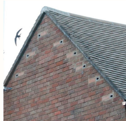
'Universal bricks' integrated within the building's fabric
