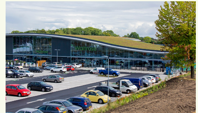
Sedum roof on Waitrose supermarket, Bagshot. Photo by Bauder UK (copyright).
